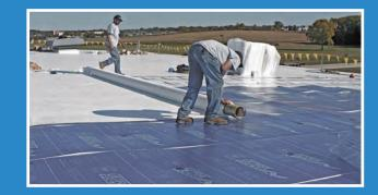
WE HOT AIR WELD ALL SEAMS. Others use adhesive which breaks down and causes leaks over time. Precise installation and heat sealing of custom pre-fabricated flashings is done around HVAC units, vents, pipes, and other protrusions on your roof.
