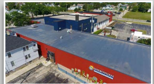
We've installed various roof colors to match Leadership Academy's overall scheme
