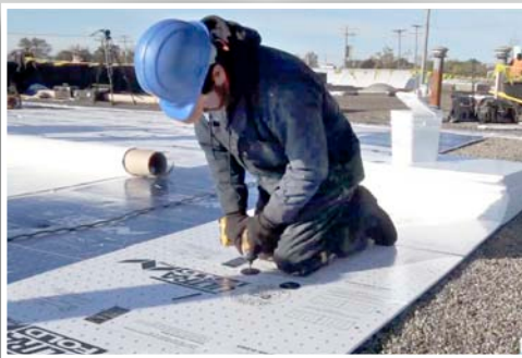
Reroofing a built-up tar roof is ideal in spring or fall.
