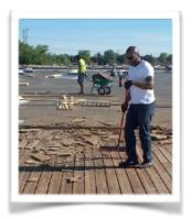
The old roof, no matter the surface, is cut and peeled off in portions. Our crew is considerate of your building and the surrounding areas below by confining removal debris to an isolated area and depositing into a dumpster.
