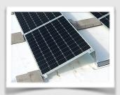
Rooftop mounted solar modules use the building's existing structure and electrical system vs. adding materials/space when installed on the ground.
