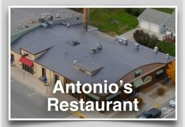
The unique rounded shape of this roof provided interesting challenges including the custom curved metal edge on the building's front which resulted in an aesthetically pleasing first-view for approaching customers. An example of what we may encounter during a reroof project: the fascia boards had to be extended and covered with sheet metal. As with all restaurants, there are lots of protrusions requiring hot air sealing of the membrane. A gray membrane vs. the more traditional white was chosen.
