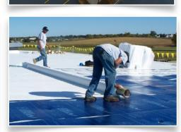
For all metal retrofit roof projects we install custom foam strips between the metal flutes and then barrier board on top to create the flat surface required for the PVC membrane.
