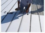
Back in 2019, we reroofed the smaller 3,200 square foot portion of the building, and this year the 8,900 square foot section by installing a PVC membrane system over the metal roof. Rust and overall deterioration of the metal made both replacements necessary.
